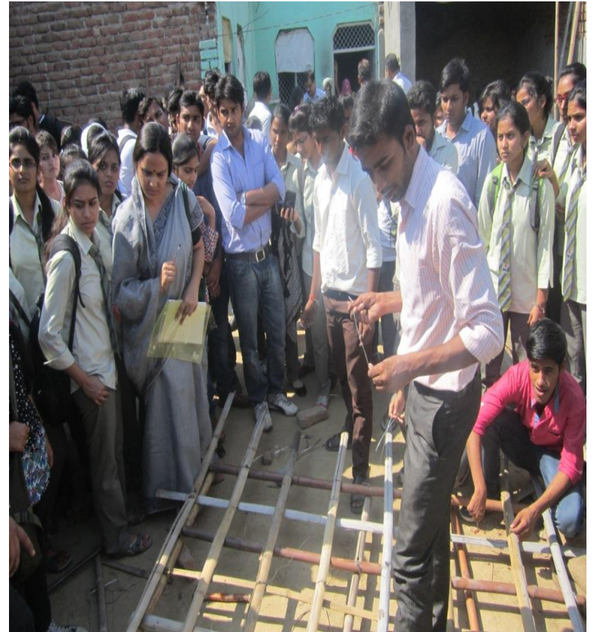
Participation of students of BE Architecture, GL Bajaj Engineering College in low cost roof construction with the help of bamboo and gunny bag for a kitchen roof top under the guidance of NITTTR, Chandigarh
