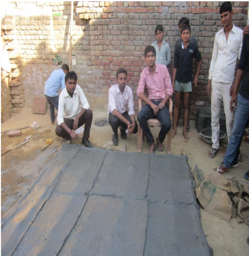
Fabrication of a Gunny Bag/Ferro-cement Roof for a Kitchen under transfer of technology by Anar Devi Khandelwal Mahila Polytechnic, Mathura at village Chaumuha, Chhatikara near Vrindavan
