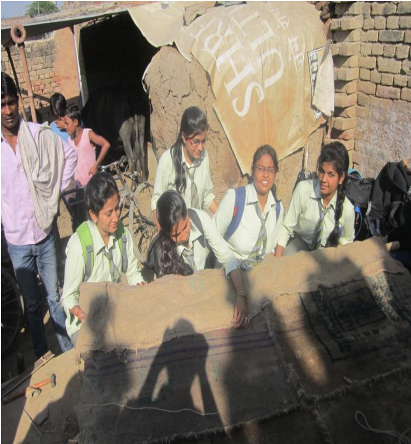
Participation of students of BE Architecture, GL Bajaj Engineering College in low cost roof construction with the help of bamboo and gunny bag for a kitchen roof top under the guidance of NITTTR, Chandigarh
